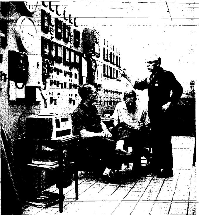
NERVE CENTER of the city power plant is this control room with its bank of instruments which tell the plant operators all they need to know about the engines producing electricity. Discussing their work are (from left) Ray Barg, Albert Anderson and Herman "Bud" Wacker. The light plant will hold open house Sunday afternoon from one to five o'clock. A special section of this issue of the paper is devoted to stories, pictures and advertisements about the light plant.
